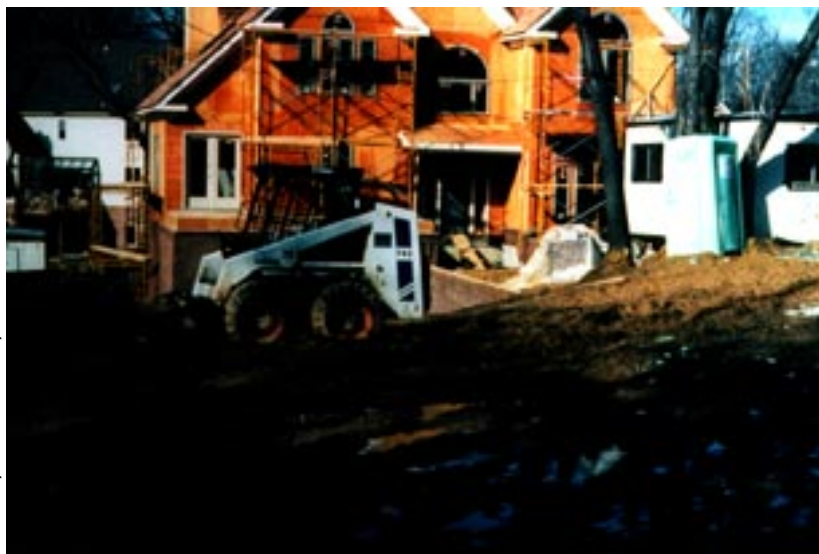
Figure 10 - The high erosion rate of construction sites is a major source of runoff from developing areas. Eroded materials contribute to siltation and eutrophication of lakes, rivers, and coastal oceans.
