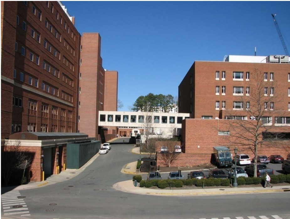
A - View of Site Location from Lane Road with South Link in foreground, Primary Care Center to the right and Jordan Hill to the left.
