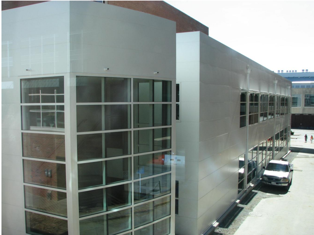
Primary Care Center Annex Occupied February 2010
