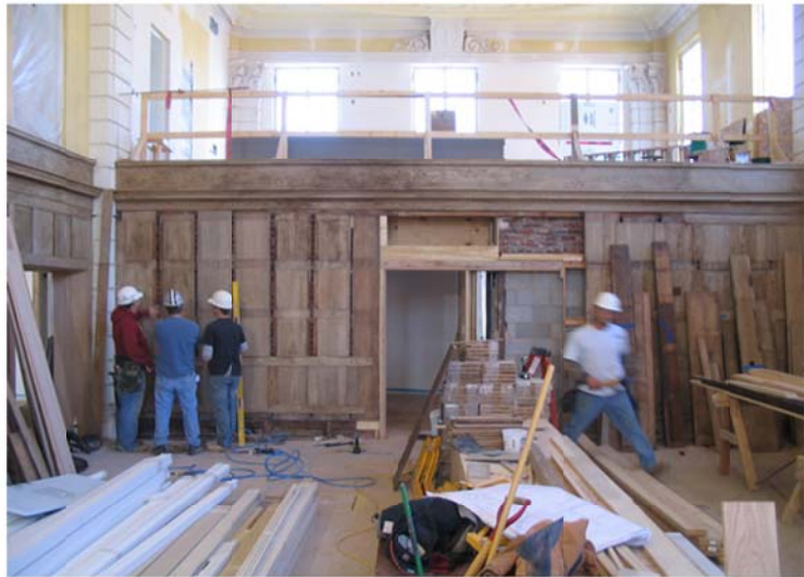
Figure 1 - Garrett Hall Renovation - Occupancy Scheduled July 2011
