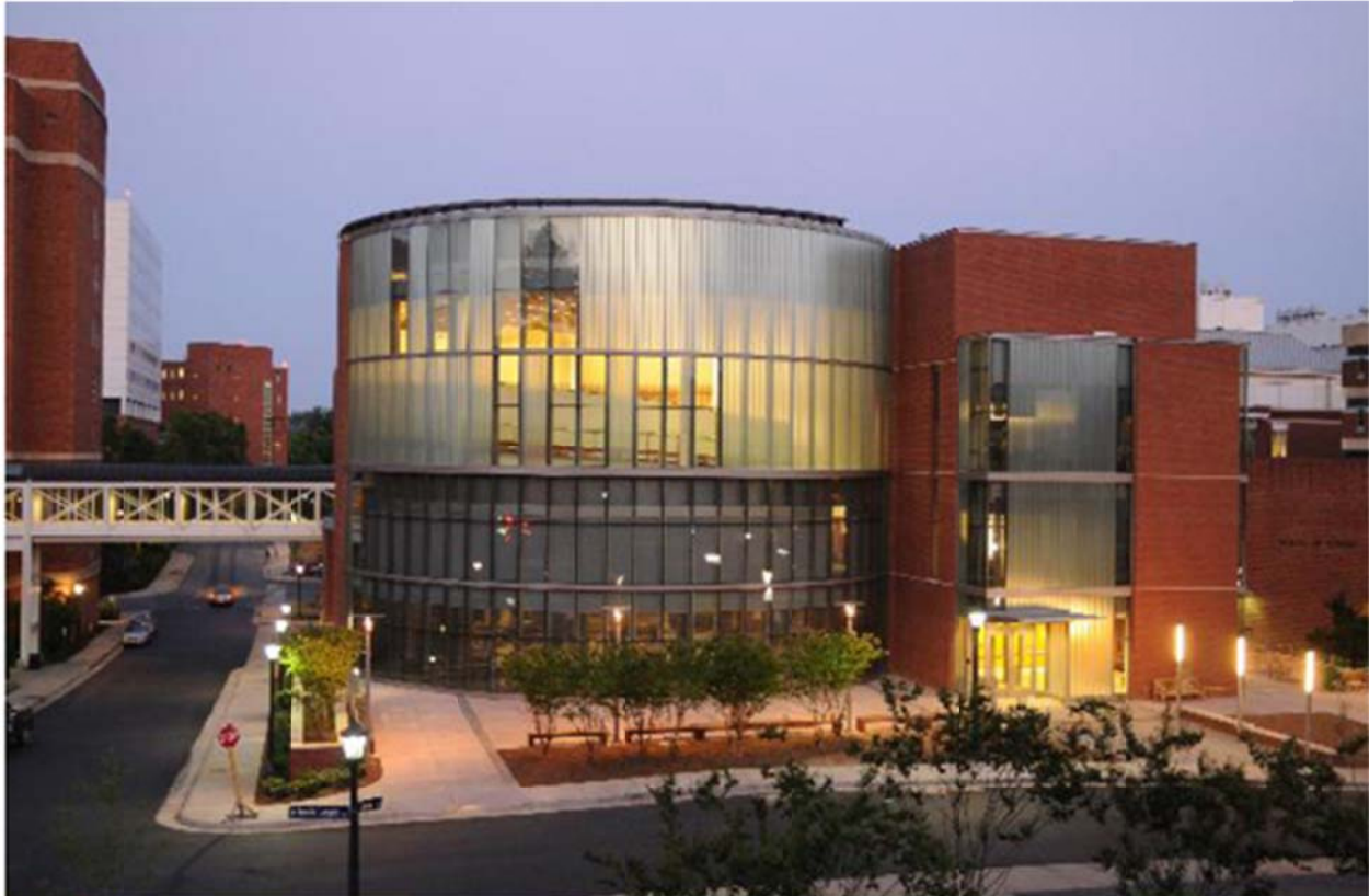
Figure 1 - Claude Moore Medical Education Building - Completed June 2010
