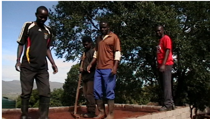
FIGURE 7 VOLUNTEERS AND AUTHORS TAMPING THE FINAL FILL LAYER
