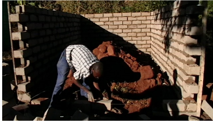
FIGURE 6 VOLUNTEER ASSEMBLING PARTIALLY BUILT WALL
